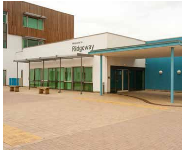
Ridgeway, Roseberry Park Hospital, Middlesbrough
